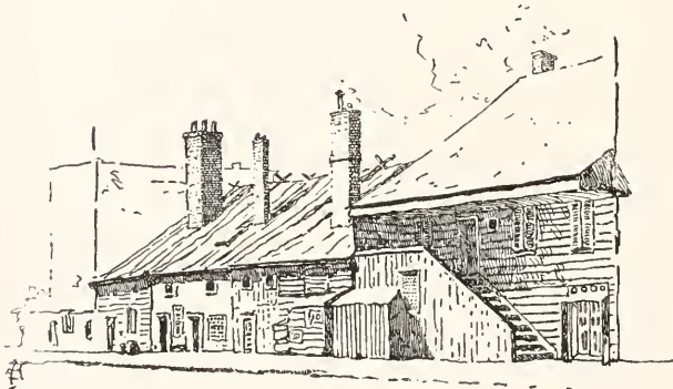
Old Houses Wiehawken St.
